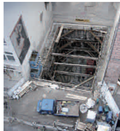
SPECIAL UNDERGROUND CONSTRUCTION
