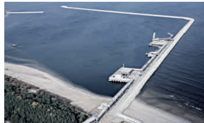
WATER AND HARBOUR CONSTRUCTION
